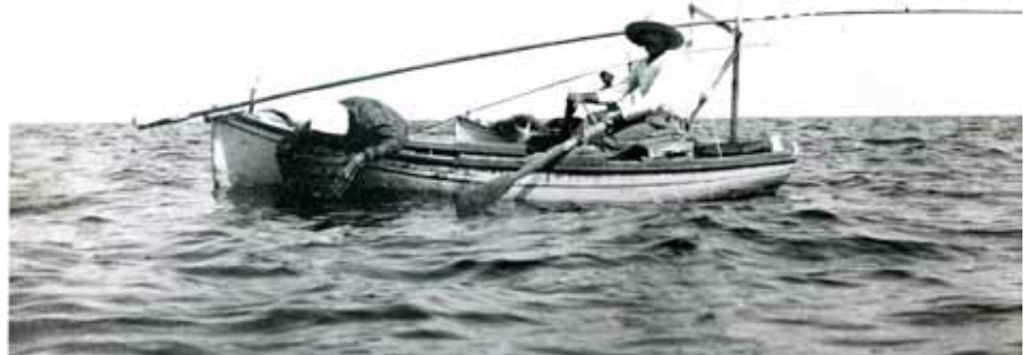
These are typical sponge dinghies at work. While one crewman looked through a glass-bottom bucket to site the sponge beds, the oarsman would locate the dinghy in the right spot. The operation had to work in water depths where the hook pole could reach the bottom. Photo courtesy of the Tarpon Springs Area Historical Society.
